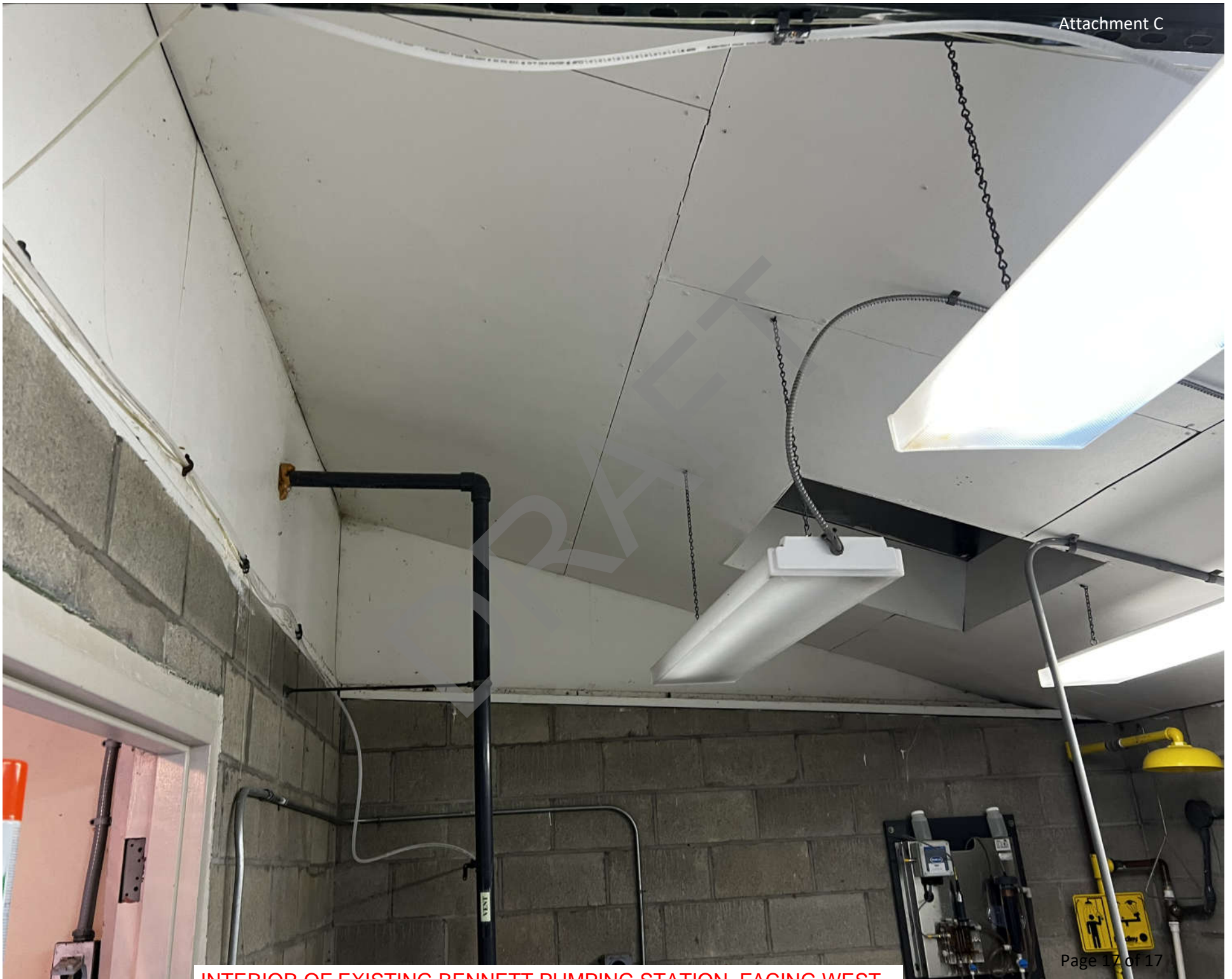
INTERIOR OF EXISTING BENNETT PUMPING STATION, FACING WEST
