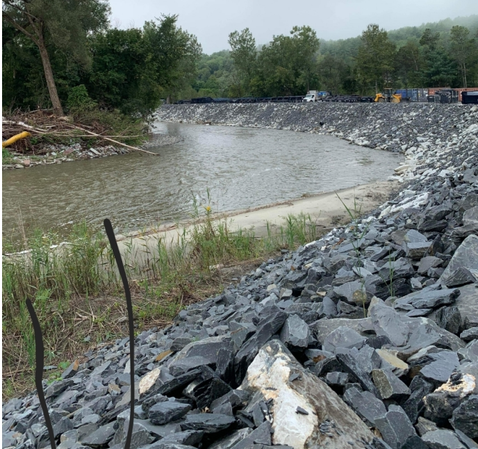
Photo of Casella flood control work provided by James Ehlers
