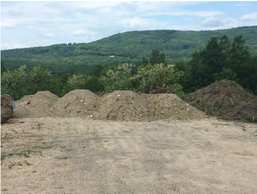
View of the 10 dump truck loads of sandy gravel fill and five dump truck loads of unscreened loam accepted by Chick's Sand & Gravel from the redevelopment of the former Littleton Sunoco facility.
