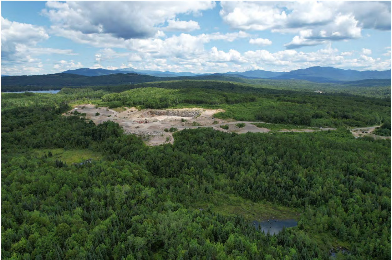
Photo 15 – Rock Quarry/Infrastructure Area Overview
