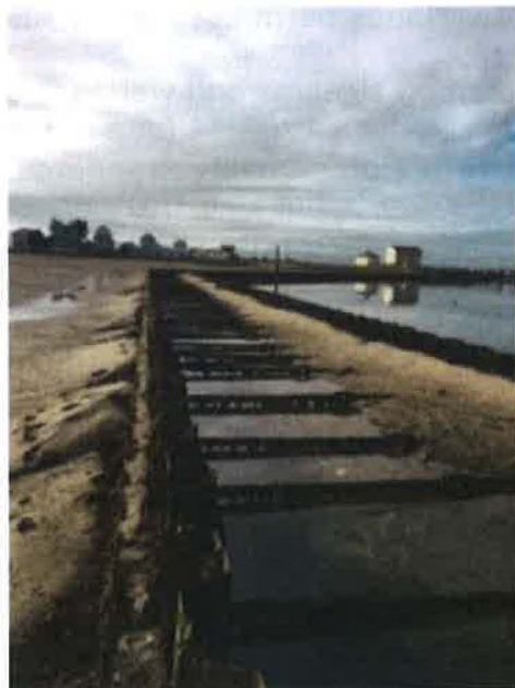
Figure 3b: Middle Ground Sediment Disposal Site- View looking south at sheet pile walls.
