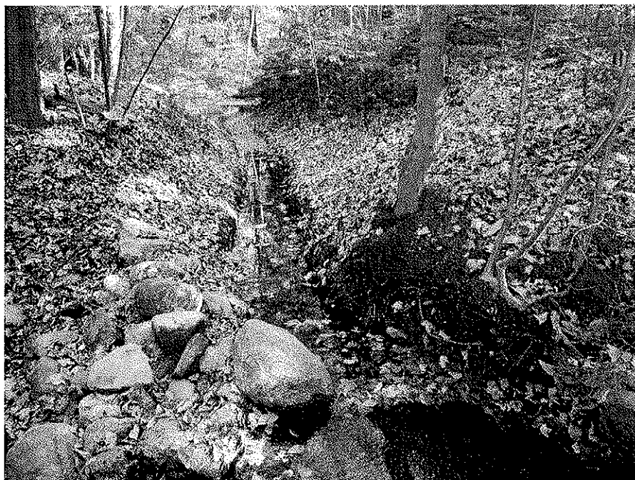
Figure 6 View looking downstream at the Chase Brook diversion ditch which conveys water from the brook to a small pool where the pump is located.
