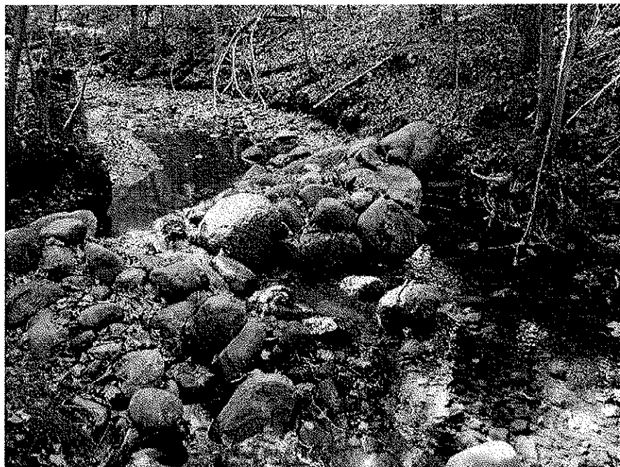
Figure 5 Chase Brook looking upstream towards the rock diversion barrier. The beginning of the diversion ditch leading to the pump pool is upstream of the rock barrier on the left.
