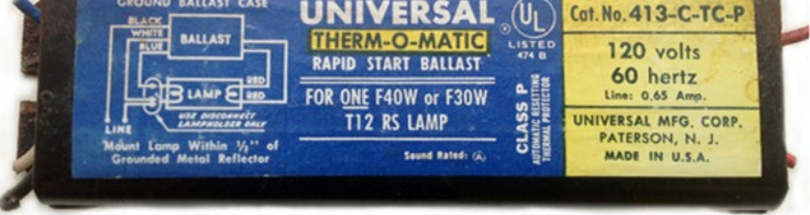
A typical pre-1979 PCB-containing fluorescent light ballast (FLB)
