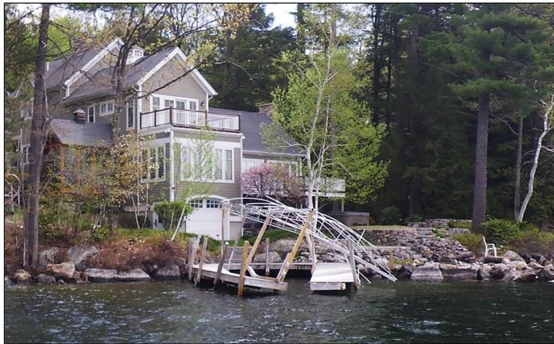
**Pictured: Existing non-tidal permanent docking structure in need of repair.**
