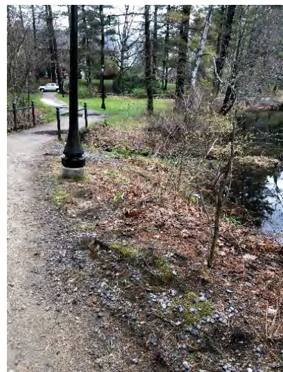
Photo 4-13: Shoreline erosion and lack of vegetated buffer.
