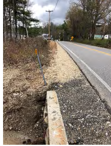
Photo 10-3: Area east of headwall.
