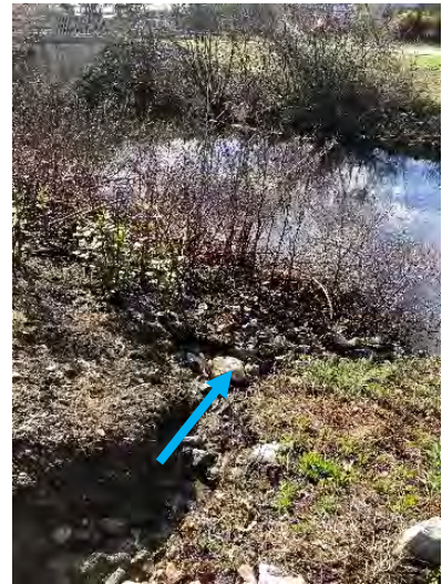
Photo 3-3: Severe erosion adjacent to water access point.
