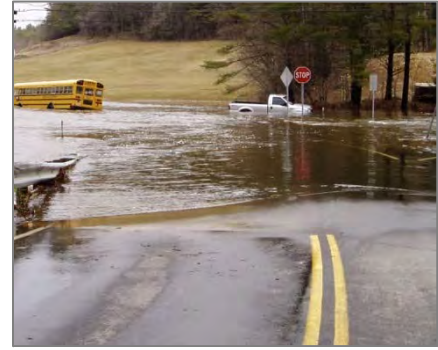
Example road flooding (Photo credit: NHDES)
