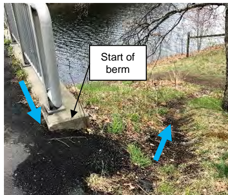
Photo 9-2: Paved drainage path leading to dirt open drainage.
