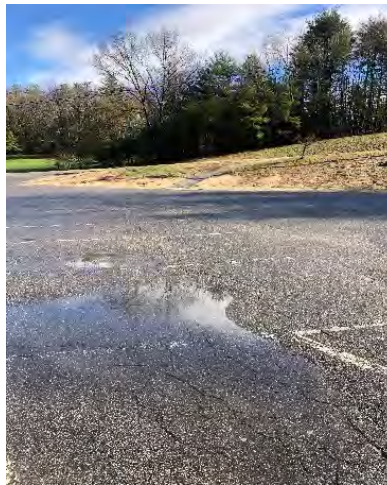
Photo 2-2: Sandy slope in north portion of parking lot, washes into catch basins.
