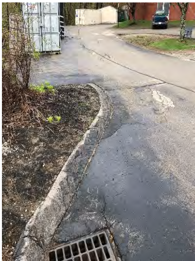
Photo 6-2: Final drainage structure before outfall.
