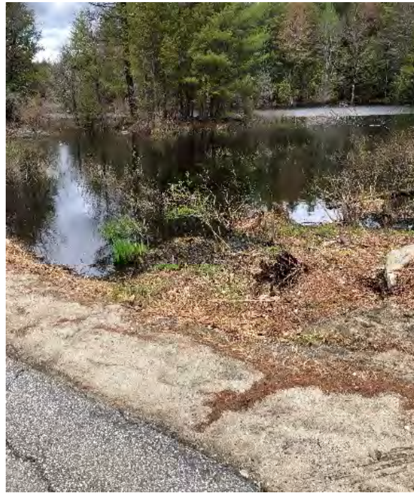
Photo 11-2: Runoff from parking area into Brook.
