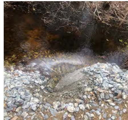
Photo 14-3: Stone surrounding culvert inlet
