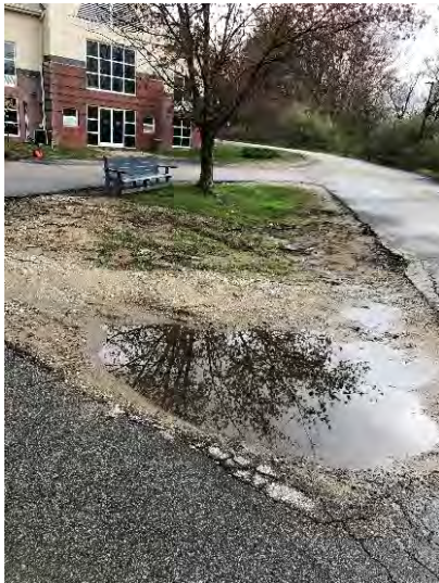
Photo 6-1: Impervious area within parking lot.
