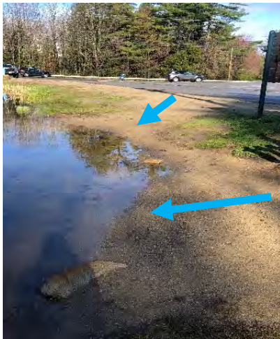
Photo 2-1: Sandy areas adjacent to parking lot wash into Bow Town Pond during rain events.
