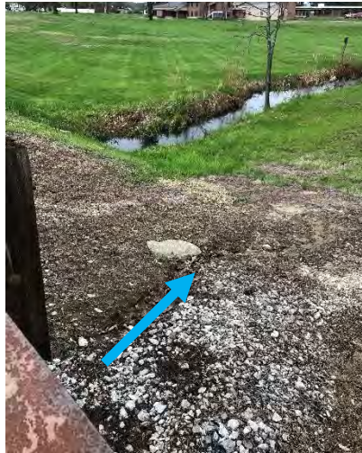
Photo 7-2: Edge of roadway erosion channel.
