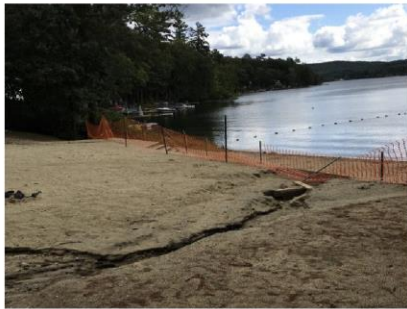
Photo taken from the 2017 Watershed BMP Assessment of Spofford Lake. This shows an area of exposed shoreline where sediments are observed as a pollutant of concern as storm water flows from the street and over the soil at the North Shore Town Beach.
