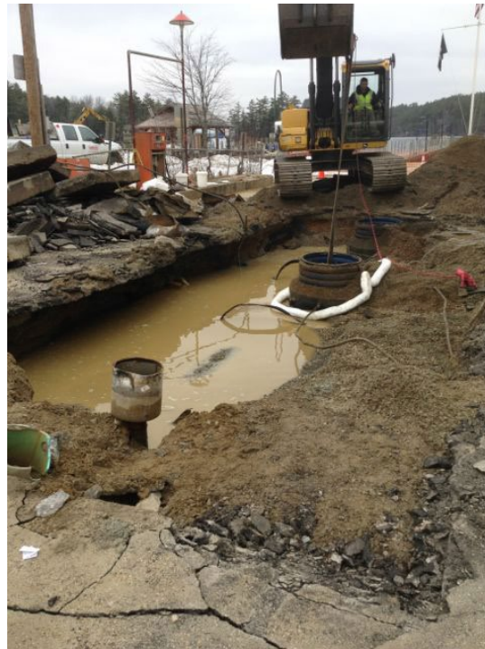
Submerged Marine Patrol Tank exposed for removal. The hold down straps were broken, and the tank was floated so that water would not get in the tank during cleaning.
