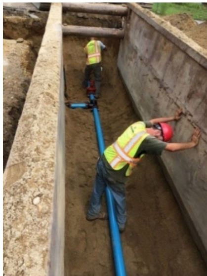
Images feature: water installation workers in a trench box; successful pressure testing of installed piping.
