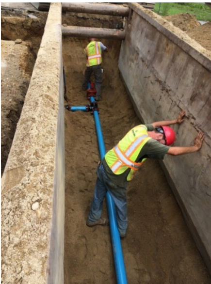
Left: Water line installation at the Little Falls Cooperative in Rochester.
