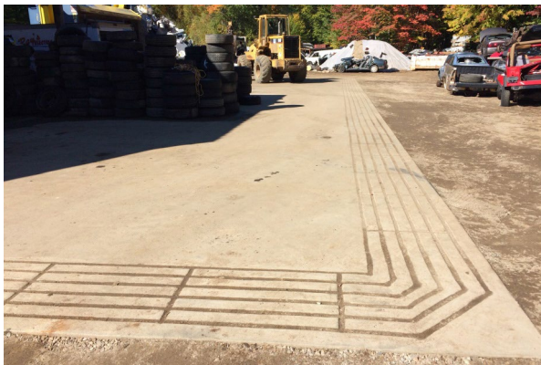
Images feature: A concrete spill-prevention pad installed by the program. Note the positive limiting barrier (PLB) in the photo. The PBL consists of grooves in the concrete designed to trap spills until they can be cleaned up; a gas buggy and fuel tank drill system being picked up by Warren's Auto Body.
