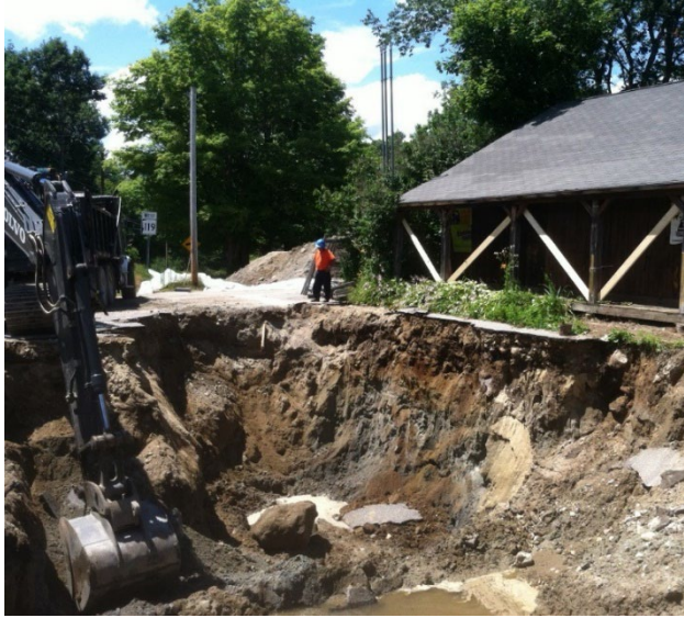
Richmond Four Corners Store contaminated soil excavation in July 2014.
