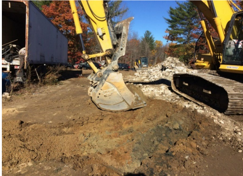
Photo of contaminated soil excavation at Epping Auto Salvage.
