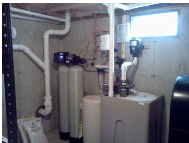
Photo of water treatment system that addresses complex MtBE contamination issue.
