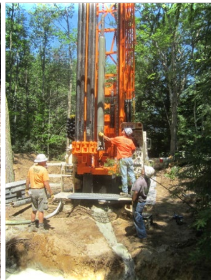
Images feature: drillers installing one of the supply wells; field technician conducting a pump test.
