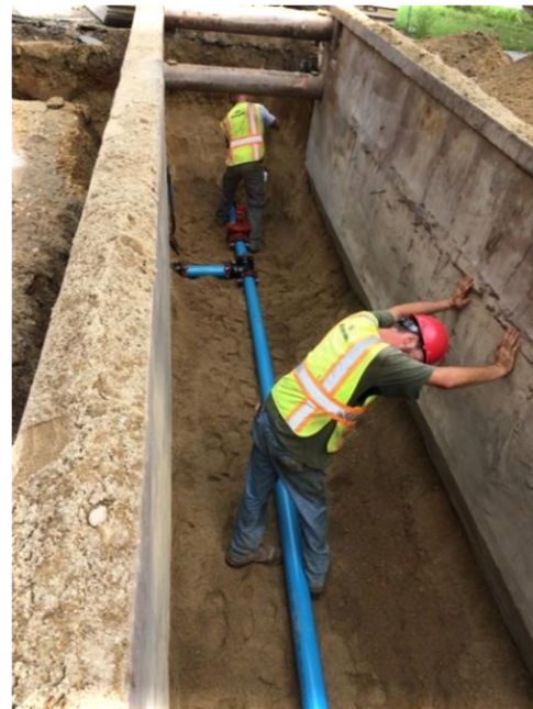
Water line installation at the Little Falls Cooperative in Rochester.
