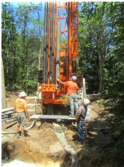
Drillers installing one of the supply wells.
