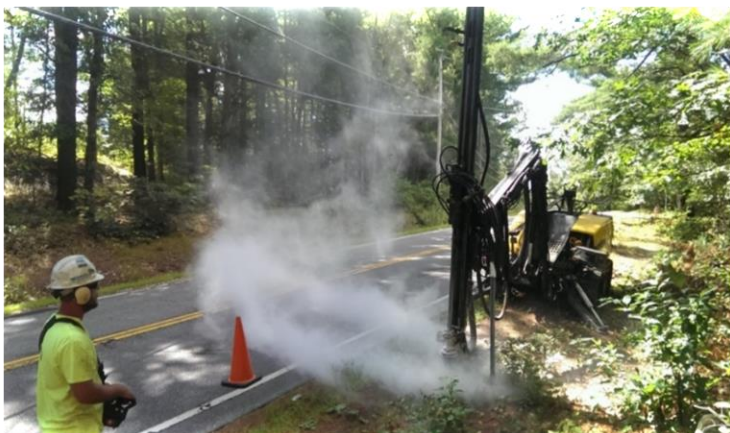
Ledge probes for the Windham water line extension.
