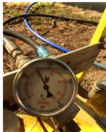
Successful pressure testing of installed piping.
