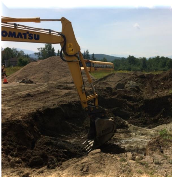
These photos show the contaminated soil being excavated.
