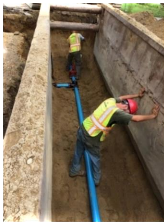
Waterline installation workers in a trench box.
