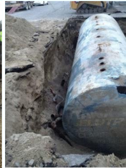
USTs prior to removal from tank graves.
