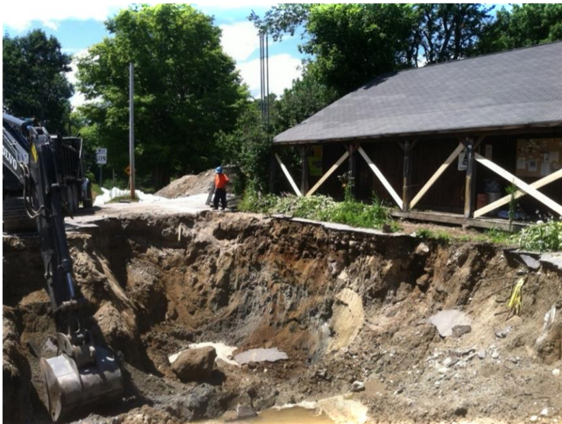
Richmond Four Corners Store contaminated soil excavation in July 2014.
