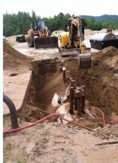
Tank top uncovered during UST removal.
