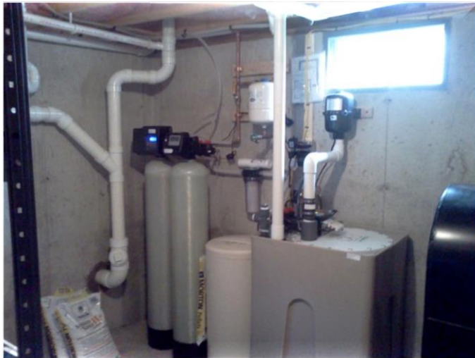
Photo of water treatment system that addresses complex MtBE contamination issue.
