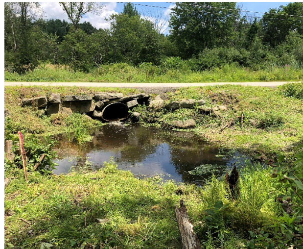
Figure 1. Culvert outlet at Bay Road and Lubberland Creek.
