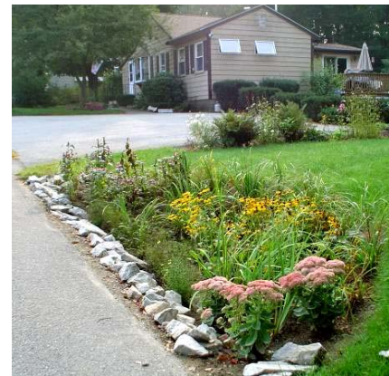
A rain garden installed on a residential property.
