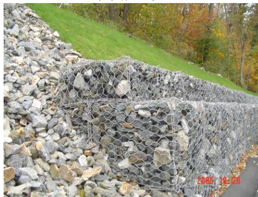
Example of gabion basket wall
