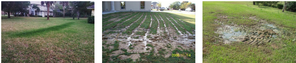
Figure 17. Examples of failing leachfields
