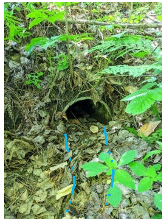
Photo 11-2: Culvert Under Hubbards Road
