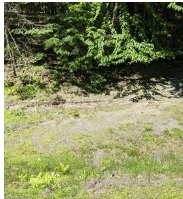
Photo 10-3: Sediment buildup in flat grassy area
