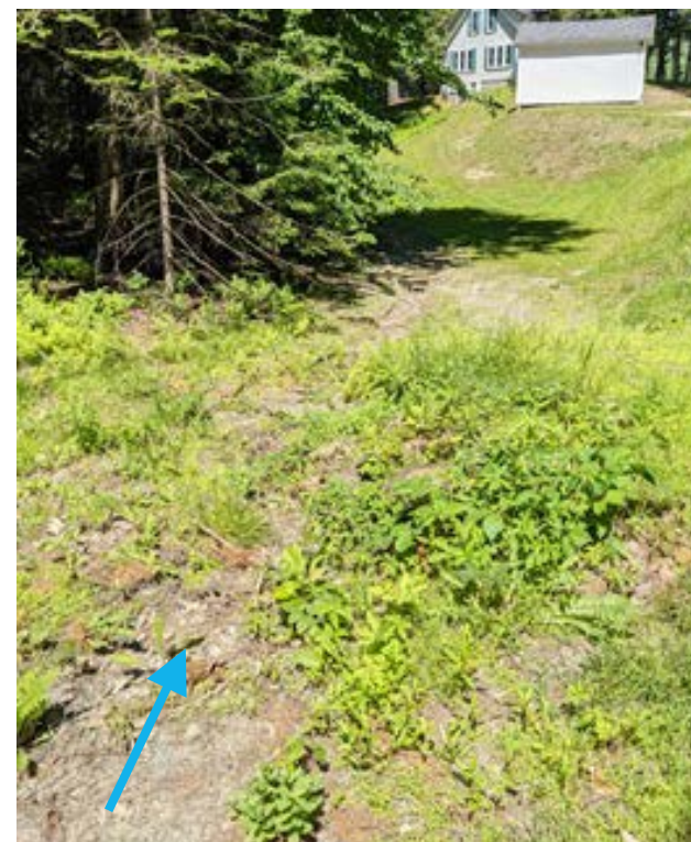
Photo 10-4: View of slope and minor erosion
