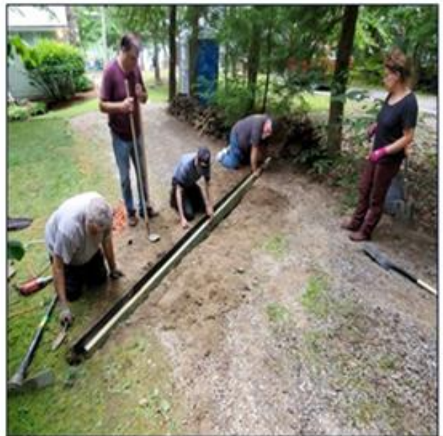
Rubber razor installation, Nippo Lake (Photo: Rob Livingston, NHDES)
