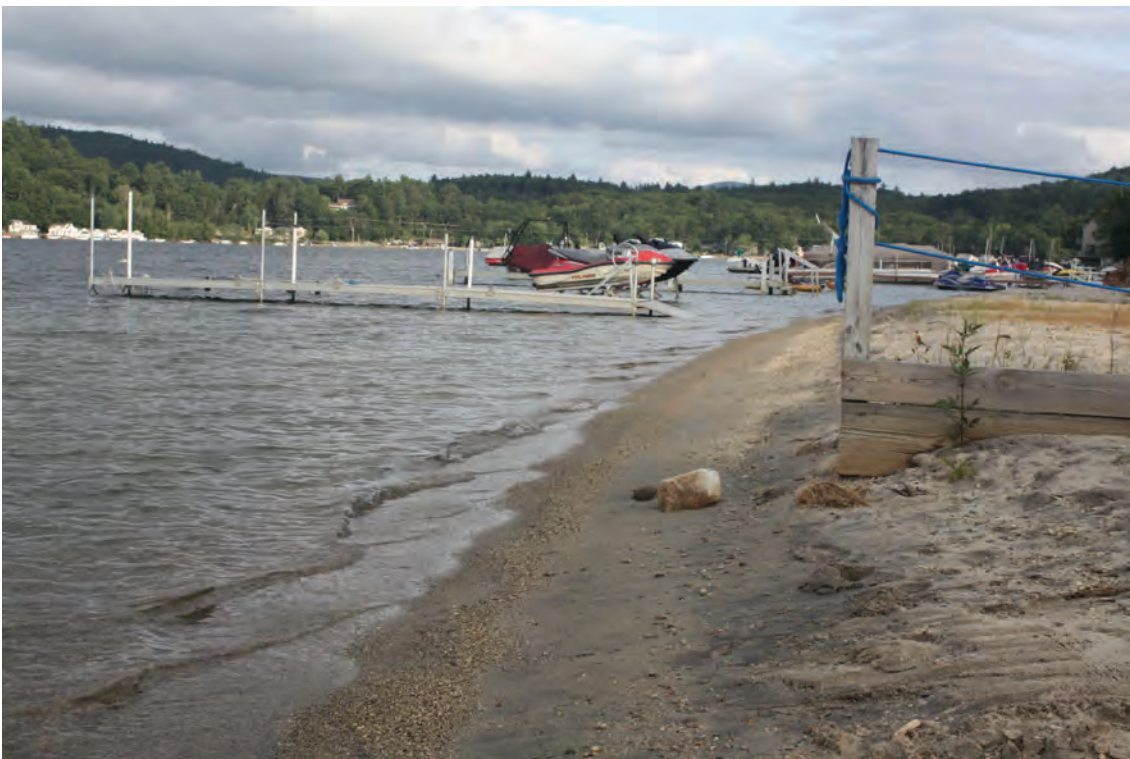
8-21-18 another view of elevation loss at other side of beach. Look at newly exposed boards on fence
