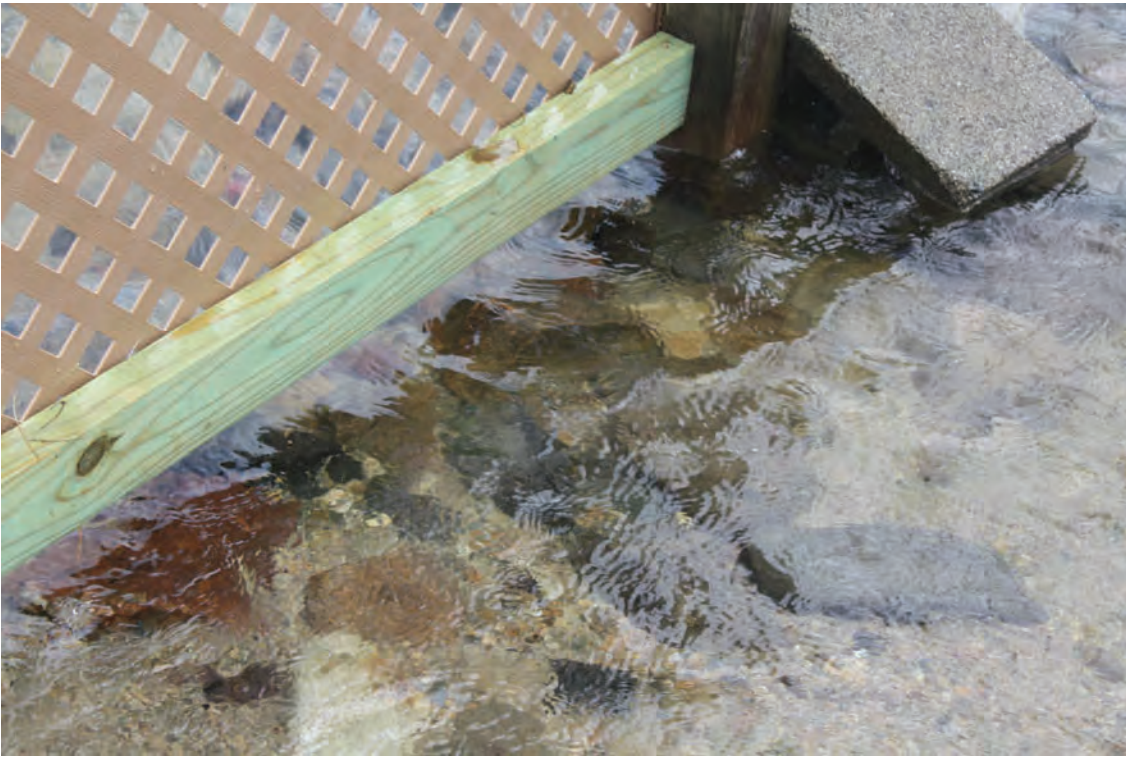
6-30-19 Rocks newly exposed due to erosion.
