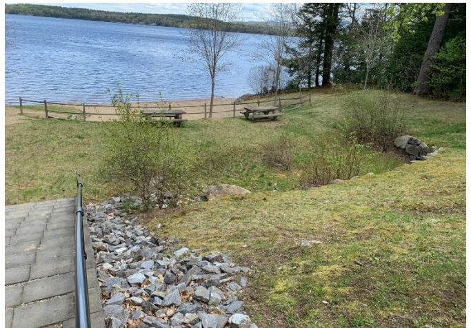
Example of structural BMPs installed at the Sanbornton Town Beach.
