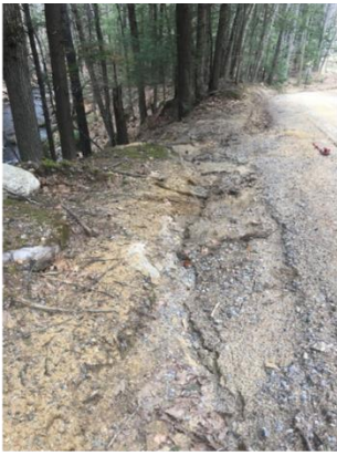
Site 1a. Lower Huse Road
