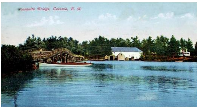
Mosquito Bridge, Laconia.
