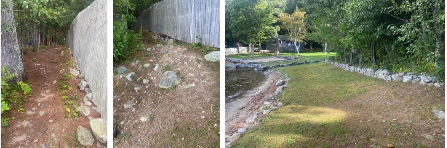
(Left) Erosion along path leading down to water, (Middle) steep area at end of path, and (Right) grass sitting/common area.
