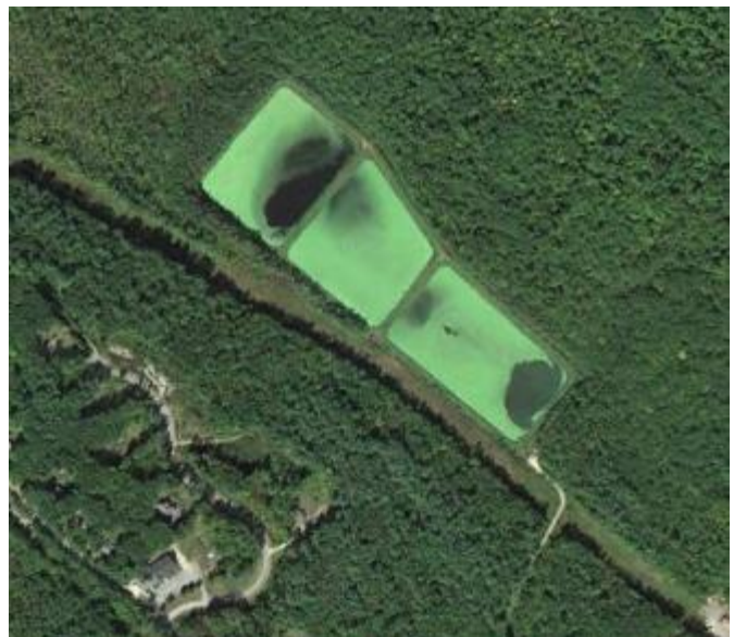
Aerial image of sewage lagoons in Moultonborough.
