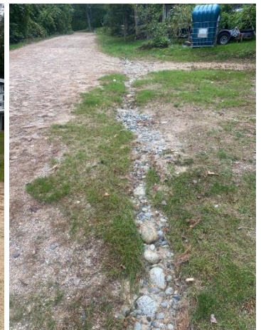
(Left) Steep grade leading directly to beach area/lake, (Right) eroded left side of road running off into gully.
