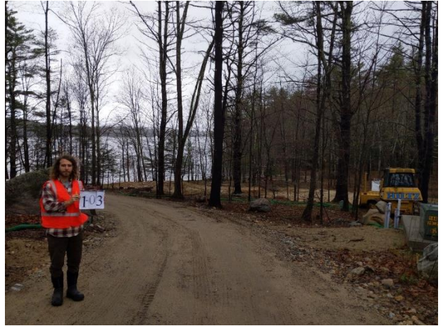
View of construction site from the top of Shady Lane.
