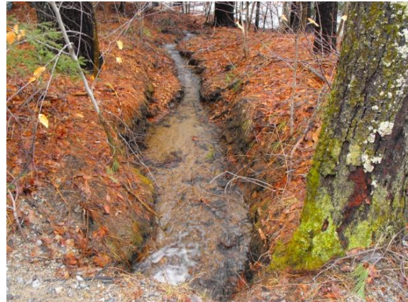
Culvert at BMP Site 18 Outlet Channel
