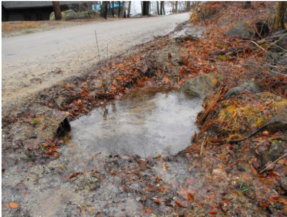
Culvert at BMP Site 18
