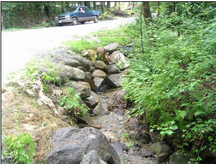
Photo 22: C18 outlet discharge to stream.
