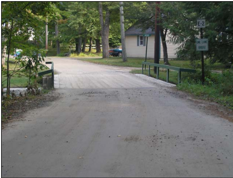
Photo 1: Bridge E-2 approach looking north.
