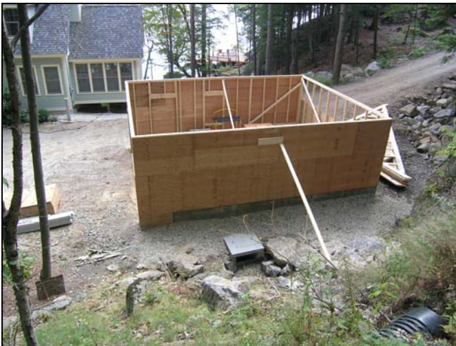
Photo 26: C22 outlet piped under garage to lake
