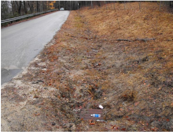
Nye Road Catch Basin (BMP Site 27)
