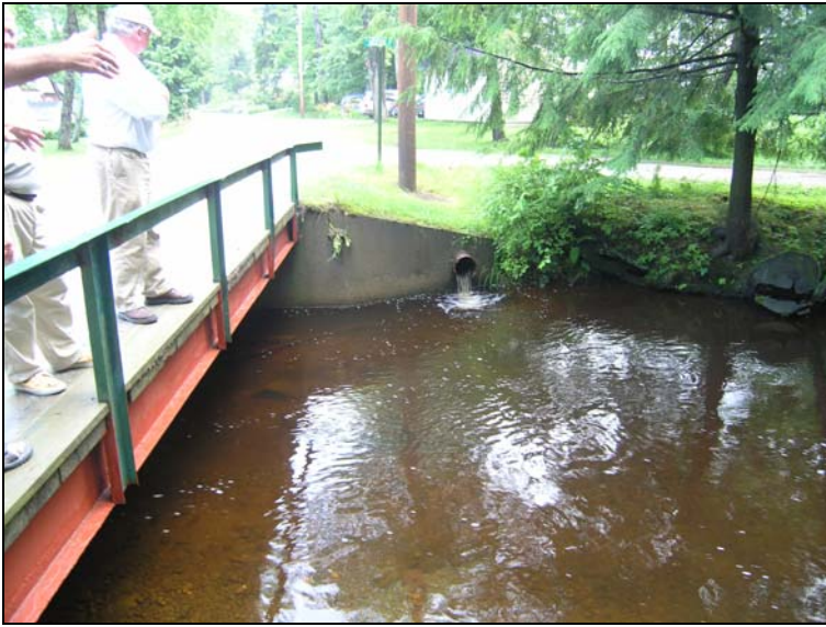
Photo 3: NE wingwall with stormwater pipe.
