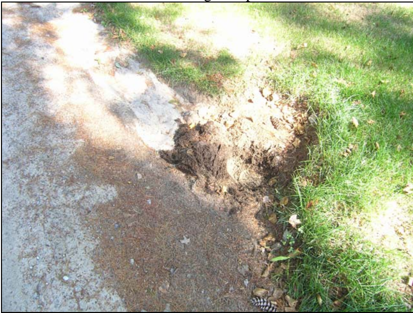
Photo 9: CB3 clogged with pine needles and sediment.
