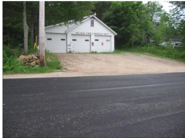
Nelson Fire Station Driveway (BMP Site 21)
