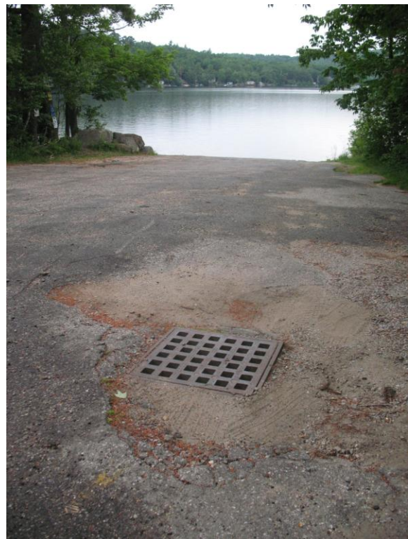
Catch Basin at Boat Ramp (BMP Site 22)
