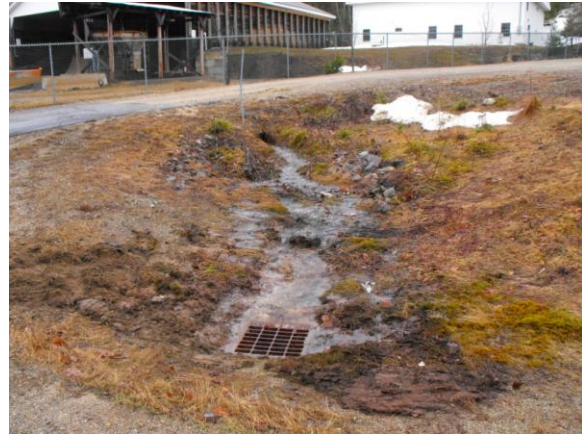
NH DOT Storage Facility Swale (BMP Site 29)
