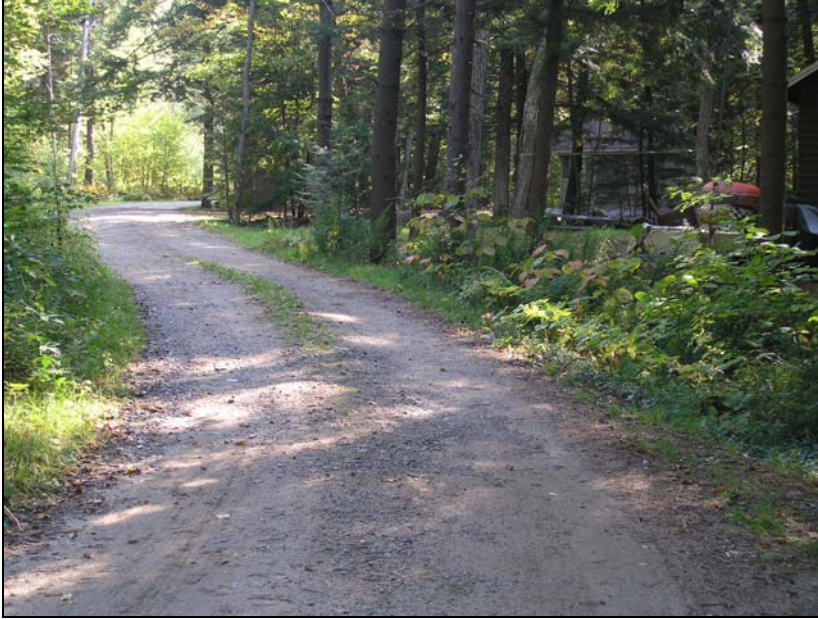
Photo 6: Jackson Road, looking East from North Shore Rd.
