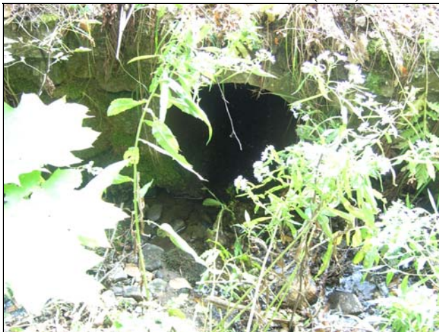
Photo 20: 24 inch concrete pipe (C16) inlet at house #564.
