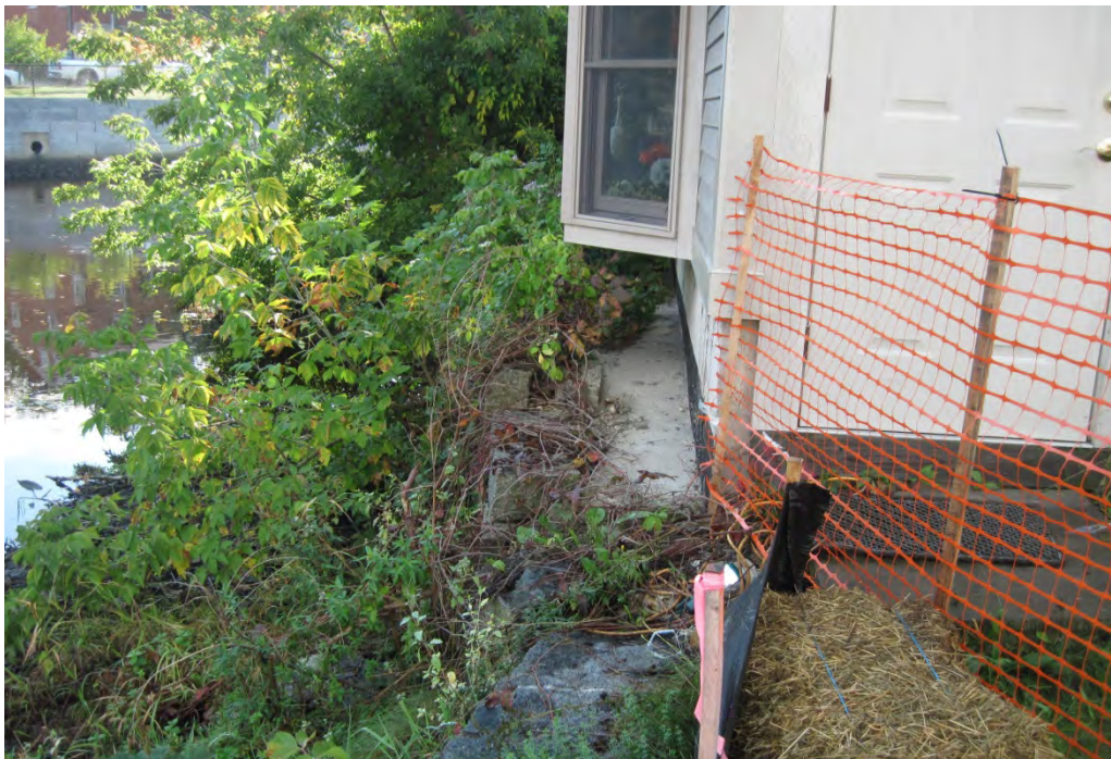
A. Concrete wall adjacent to foundation wall
