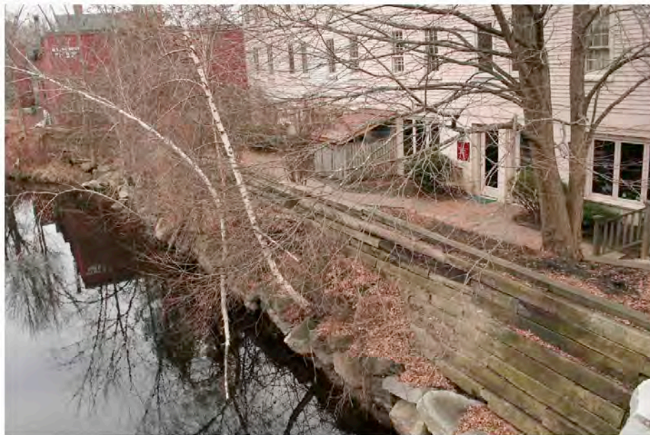
B. Upstream of Great Bridge – The banks are protected by a) rock walls and b) retaining walls
