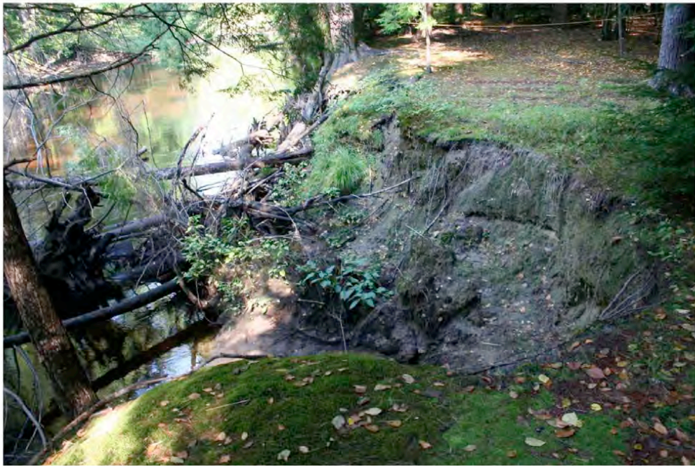
A. A view of bank slumping located west of the Amtrak Railroad Line, beyond the upper limit of the impoundment. This type of slumping may become more prevalent in the impoundment area following dam removal. (See Figure 3.3-1 for photo location.)
