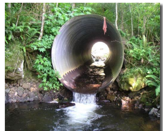
An undersized culvert ranked as “fully incompatible” that has significant downstream bed scour and bank erosion.
