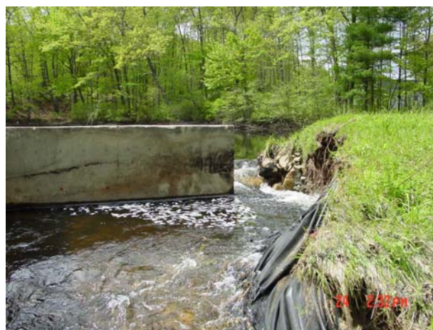
Breach of Noyes Pond Spillway
