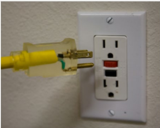
Level 1 Charging - Standard House Outlet
