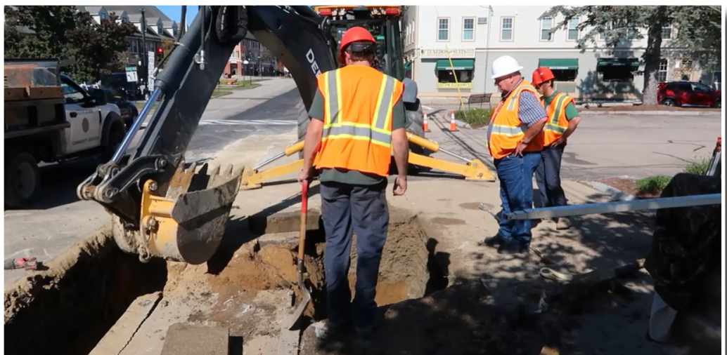
Installation of a tree box stormwater filter in the city core.
