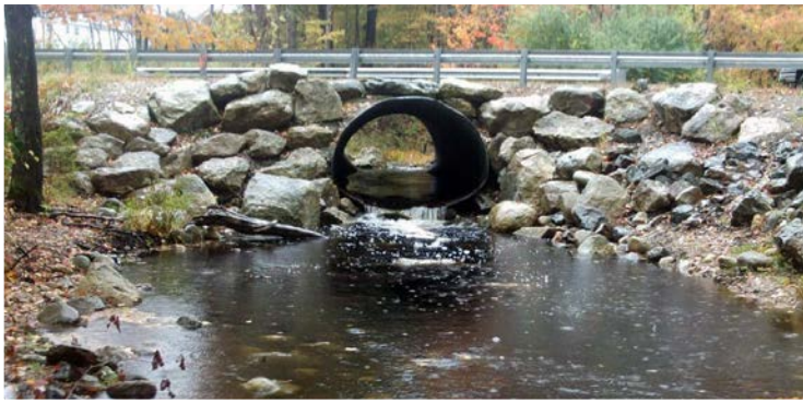
Oyster River perched culvert. Image credit: The Nature Conservancy
