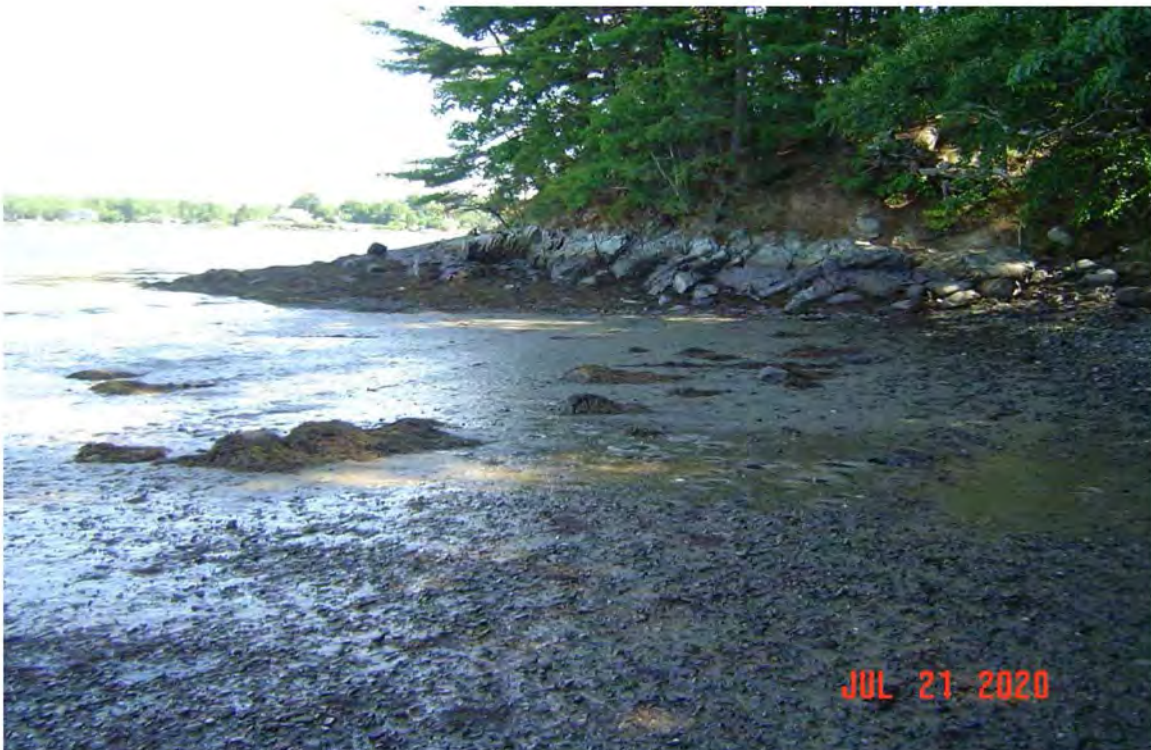
Image 8 – Looking north at low tide from atop the existing line water line (and the location in image 7 above) in Newington. (©Jacobs2020)
