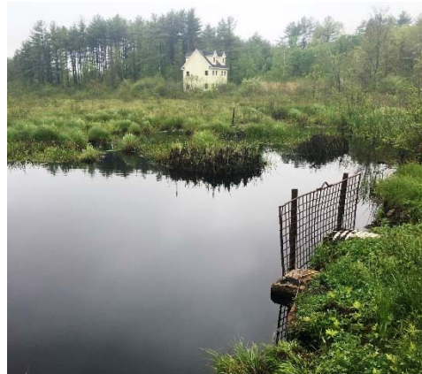
Upstream side of Winnicut River at Lovering Road culvert
