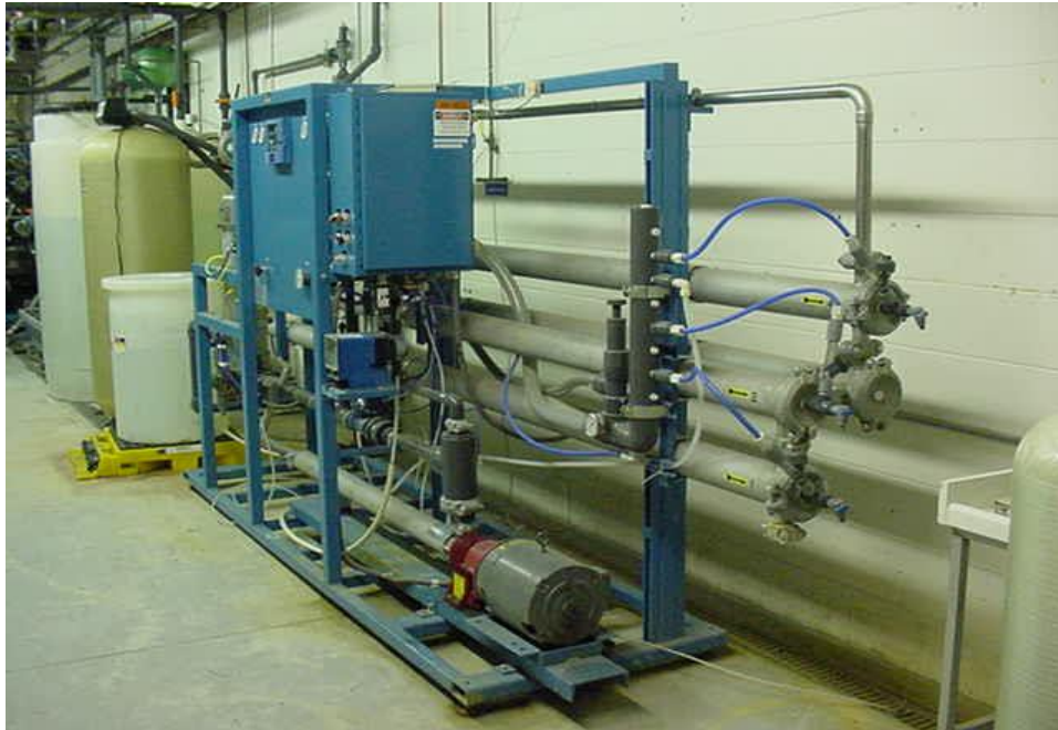
Photo 3. Millipore's R/O Unit #3 (Storage Tank #3 and Carbon/UV treatment system in the background)
