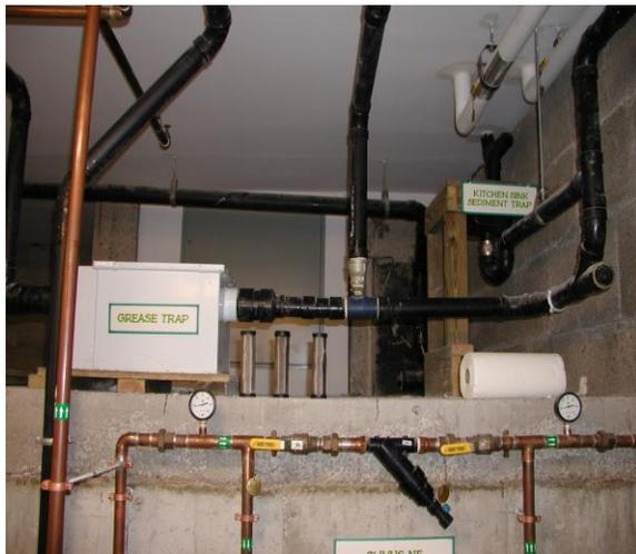
Photo 8. Sediment and grease traps
