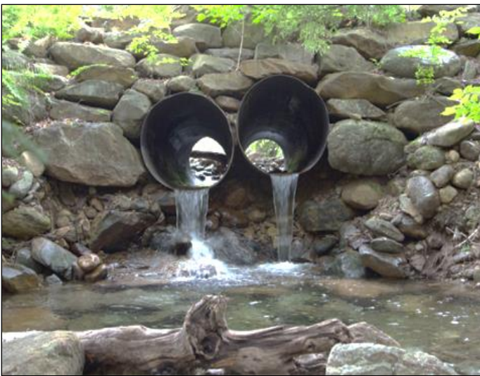
Figure 4 – The twin perched culverts shown on the left were replaced with the fully-spanning stream crossing shown on the right, which provides geomorphic compatibility and adequate hydraulic capacity, as well as allowing aquatic organism passage.
