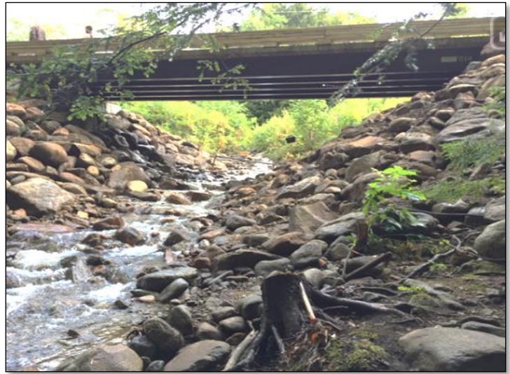
Figure 4 – The twin perched culverts shown on the left were replaced with the fully-spanning stream crossing shown on the right, which provides geomorphic compatibility and adequate hydraulic capacity, as well as allowing aquatic organism passage.
