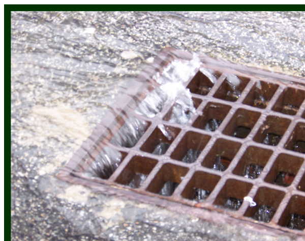
Stormwater flows into a catch basin from a commercial parking lot during a rainstorm in Concord, New Hampshire.
