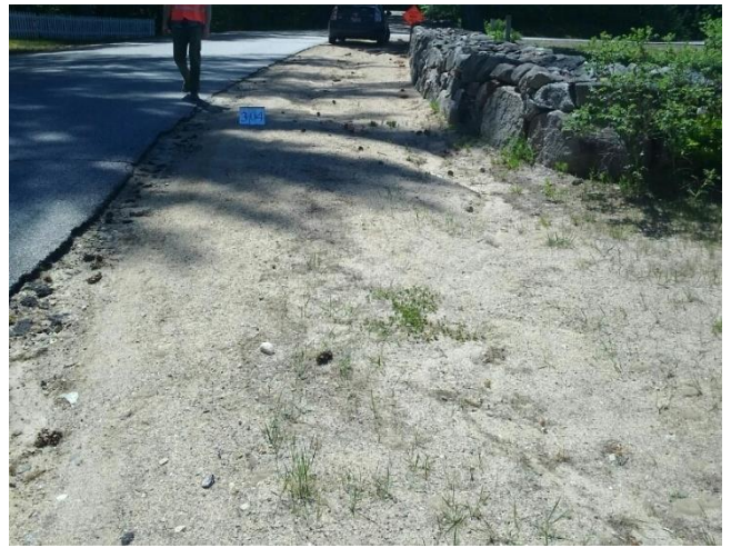
Site 3-04: Intersection of East Holderness Rd and Rt. 3
