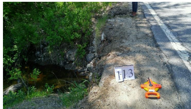
Site 1-13: Road crossing on Rt. 175 by house #421.
