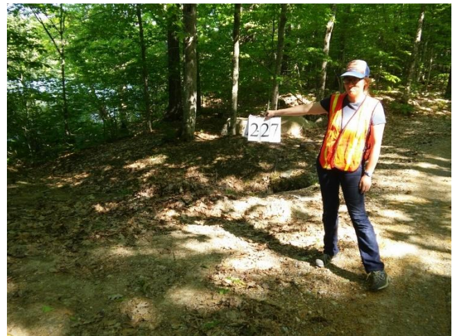
Site 2-26: Metcalf Rd, cross-culvert (note incorrect site label in photo).
