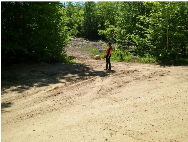
Site 2-10: Thompson Rd.
