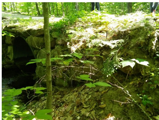
Site 2-27: Metcalf Rd, cross-culvert.
