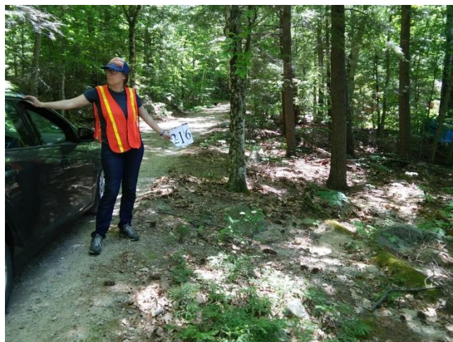
Site 2-16: Intervale Pond Rd, road wash-out.
