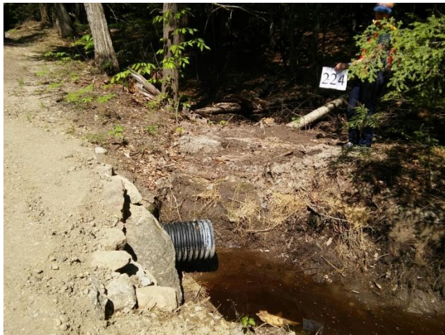
Site 2-24: Coolidge Farm cross-culvert.
