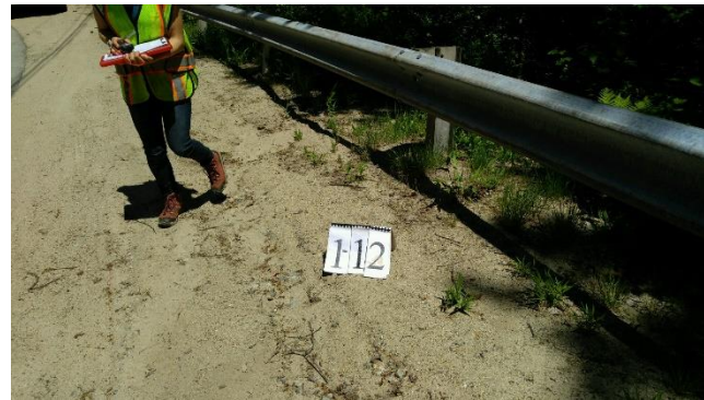
Site 1-12: Road shoulder by house #296 Beede Rd.
