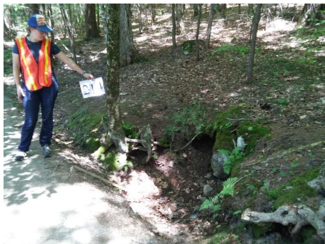
Site 2-14: Intervale Pond Rd cross-culvert.
