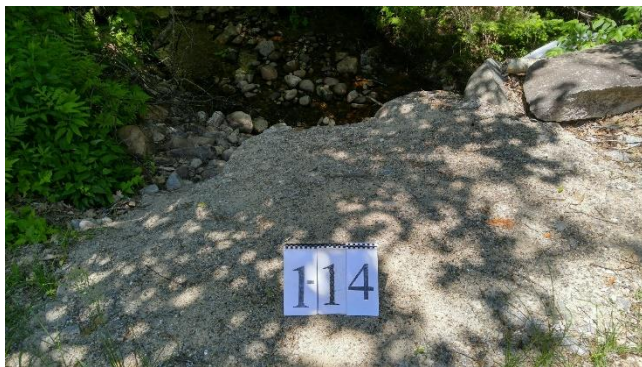
Site 1-14: Road crossing on Beede Rd (Carr Brook).
