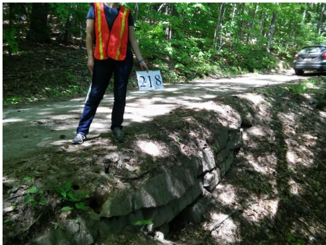
Site 2-18: Jimmy Point Rd, stone culvert.
