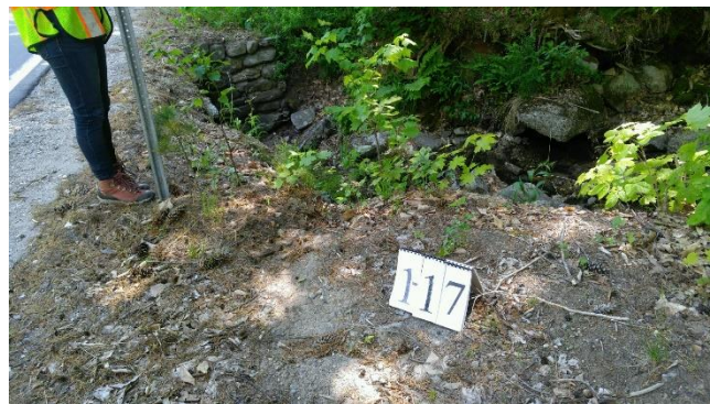
Site 1-17: Road crossing on Rt. 113 (West Brook).
