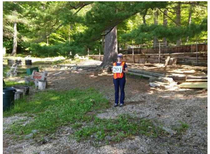
High use impact generating uncontrolled stormwater runoff at Camp Hale.
