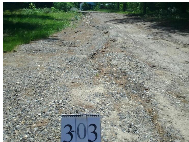
Site 3-03: Rt. 3 driveway before Owl's Landing Campground.
