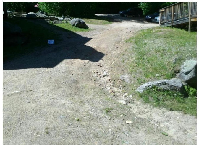
Steep gravel driveway of Squam Lakes Association's crew cabin causing significant gully formation.
