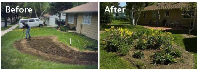
Rain Gardens are often effective residential BMPs for treating stormwater on-site.
