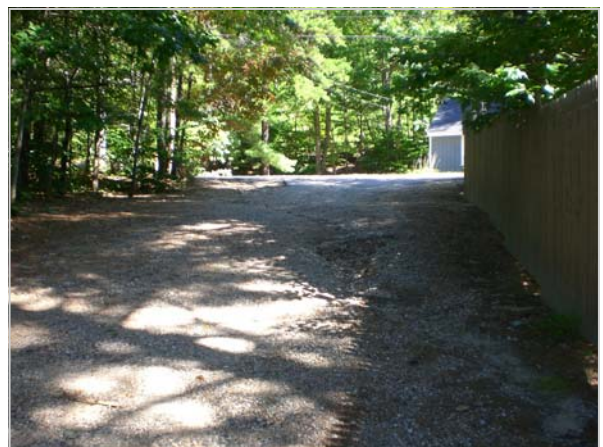
Signs of erosion were noted near the Lake Ivanhoe boat launch.
