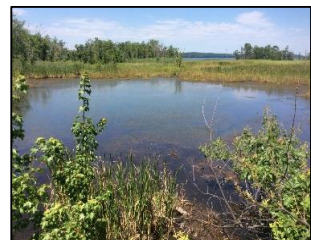
DS view above structure
