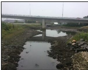
DS view above structure
