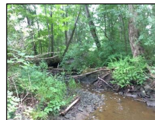
DS view above structure
