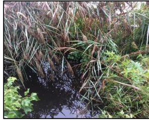
DS view toward structure
