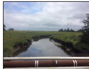
DS view above structure
