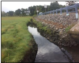
DS view above structure
