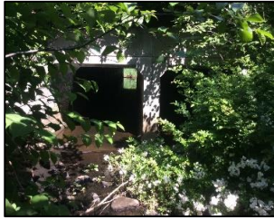
DS view toward structure
