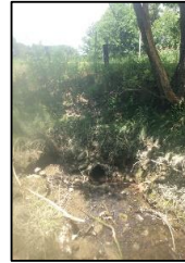
DS view toward structure
