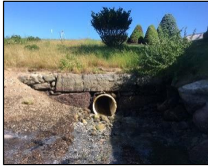
DS view toward structure
