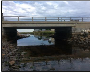
DS view toward structure
