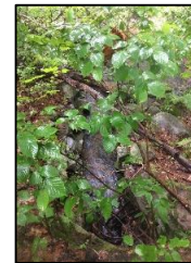
DS view above structure
