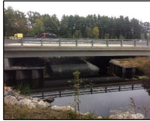
DS view toward structure
