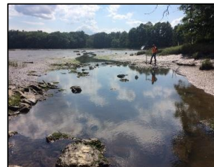
DS view above structure
