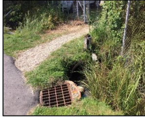
DS view toward structure
