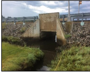
DS view toward structure
