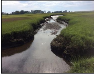
DS view above structure
