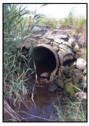
DS view toward structure
