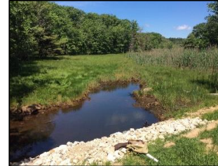
DS view above structure
