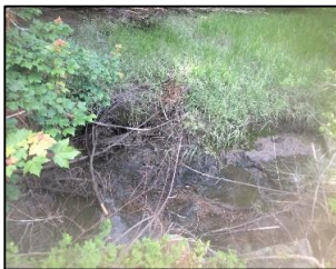
DS view above structure
