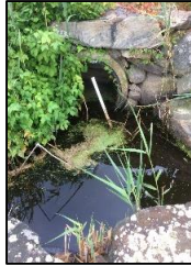
DS view toward structure
