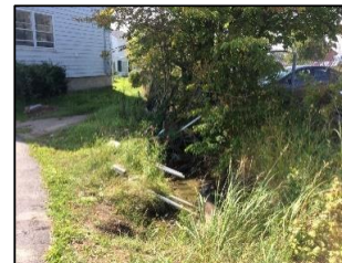
DS view above structure
