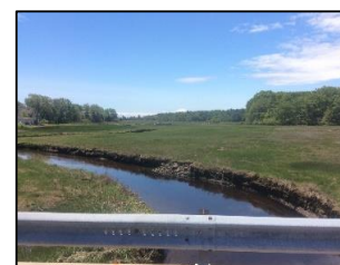
DS view above structure
