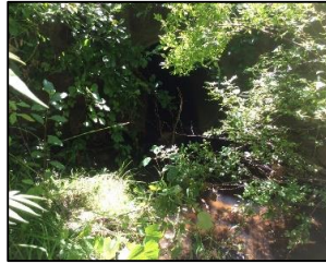
DS view toward structure
