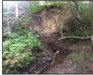
DS view toward structure
