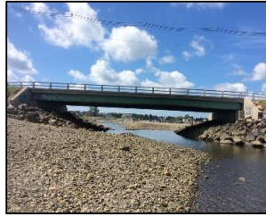
DS view toward structure
