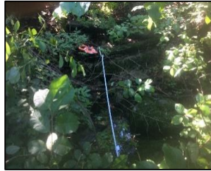
DS view toward structure
