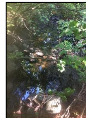
DS view above structure
