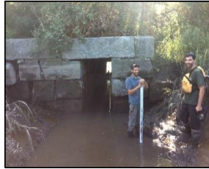
DS view toward structure
