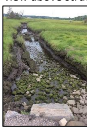
DS view above structure
