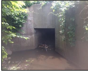
DS view toward structure
