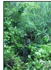
DS view above structure
