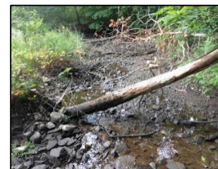
DS view above structure
