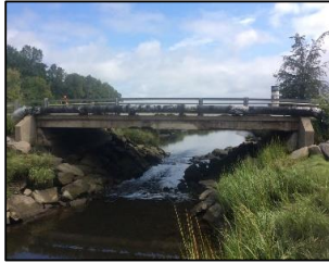
DS view toward structure
