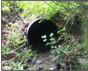
DS view toward structure
