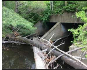
DS view toward structure
