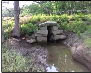
DS view toward structure
