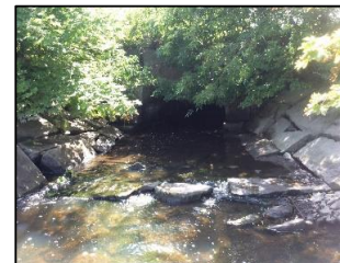
DS view above structure
