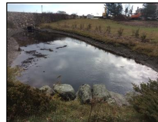
DS view above structure
