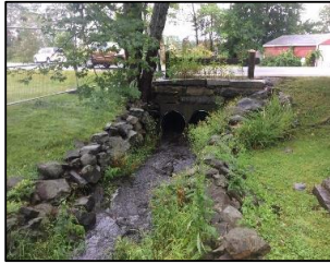
DS view toward structure
