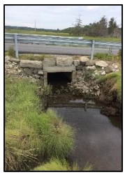
DS view toward structure
