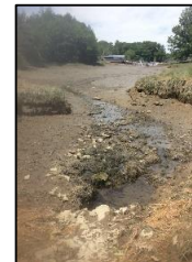
DS view above structure
