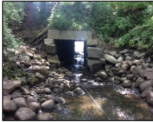
DS view toward structure
