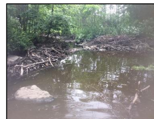
DS view above structure
