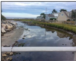
DS view above structure
