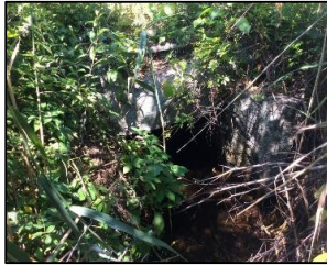
DS view toward structure
