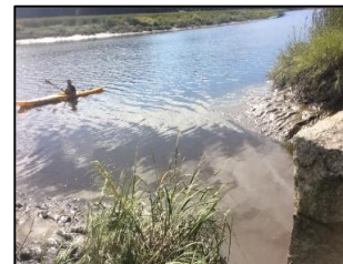
DS view above structure
