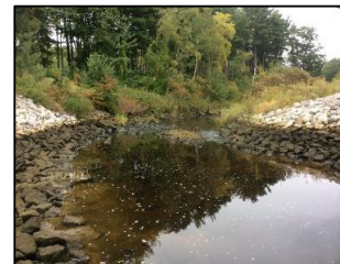
DS view above structure
