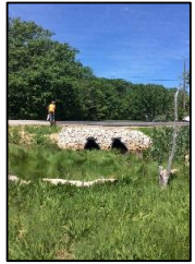
DS view toward structure
