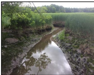
DS view above structure
