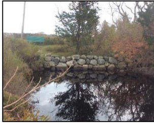
DS view toward structure
