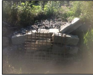
DS view toward structure
