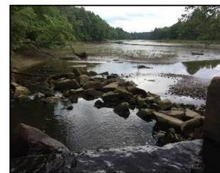
DS view above structure
