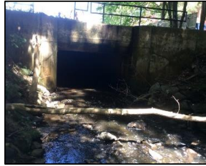
DS view toward structure
