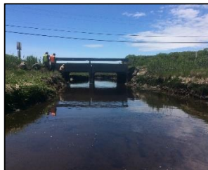
DS view toward structure
