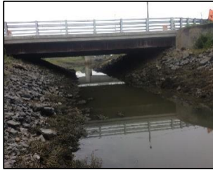
DS view toward structure
