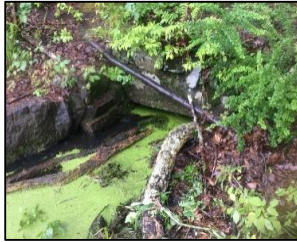
DS view toward structure
