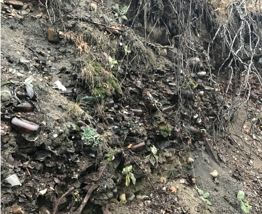
Figure 3. The eroding bank of the river showing materials from the landfill. The bank is very unstable – and undercut.
