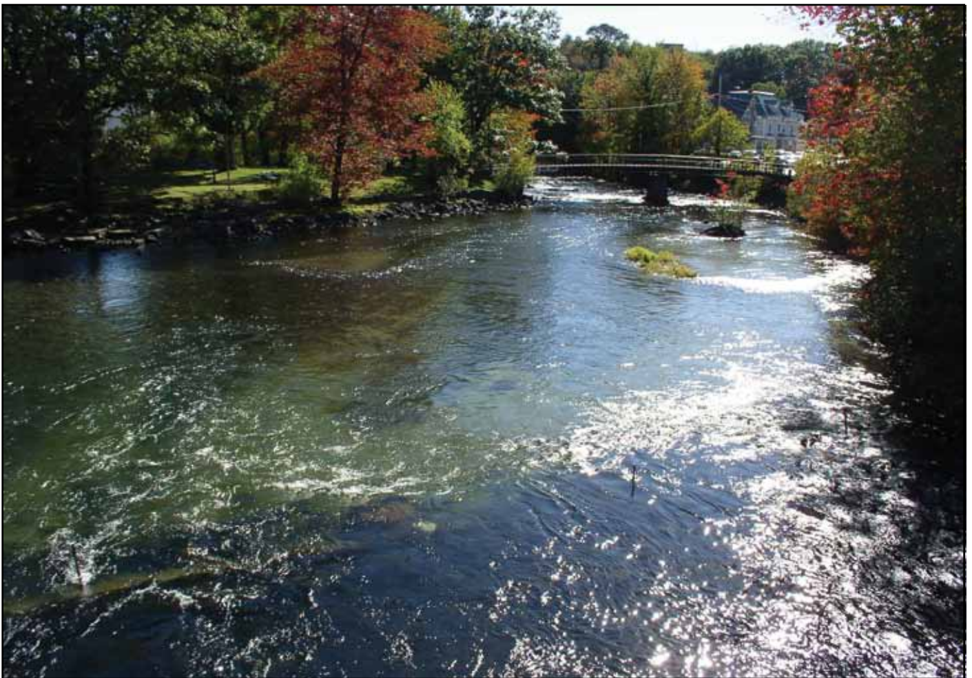
Directional drilling technology facilitates the replacement of water mains such as the one crossing the Winnepesaukee River.
