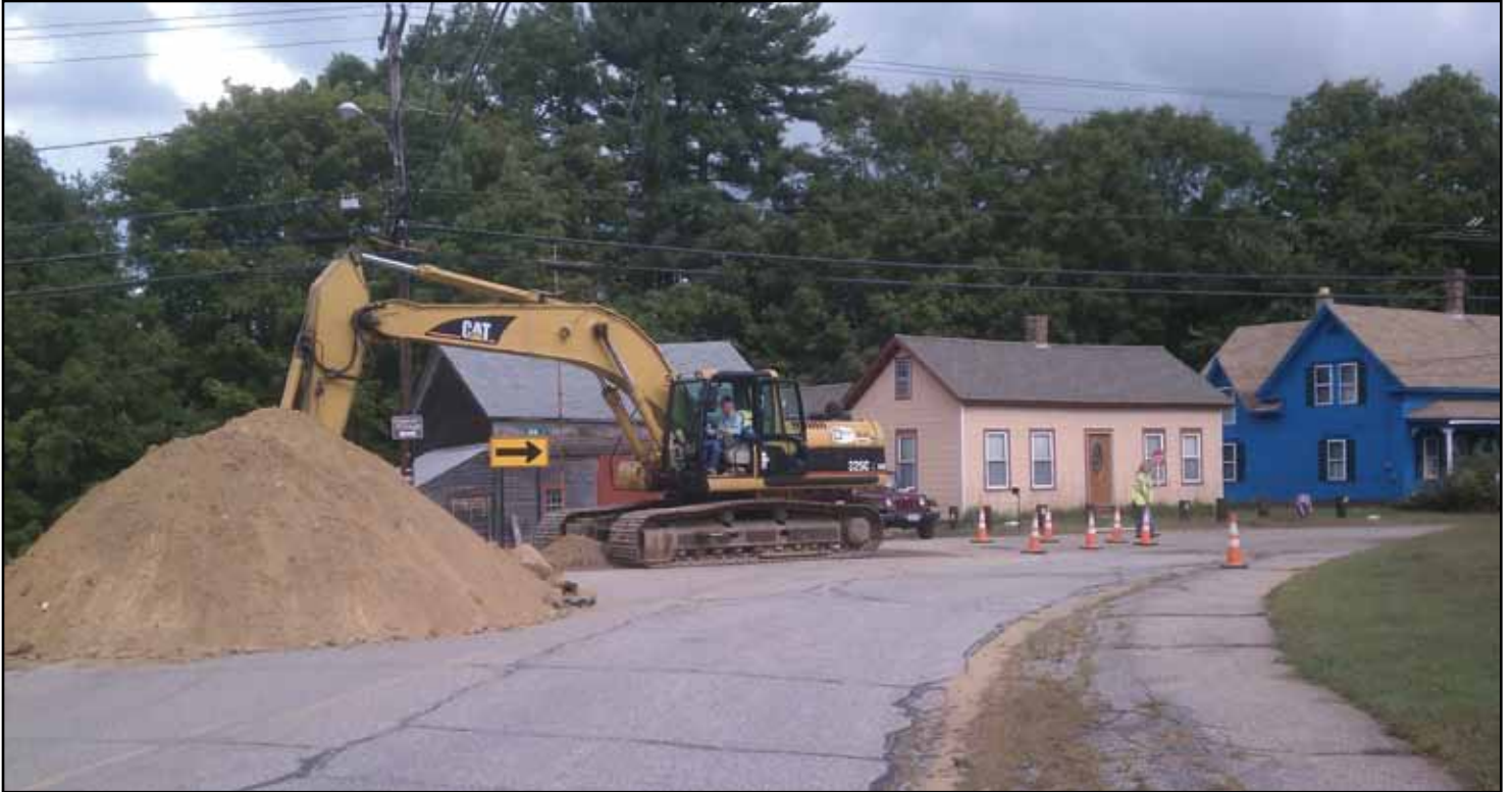
Excavation begins to replace the aging water mains in downtown Belmont.
