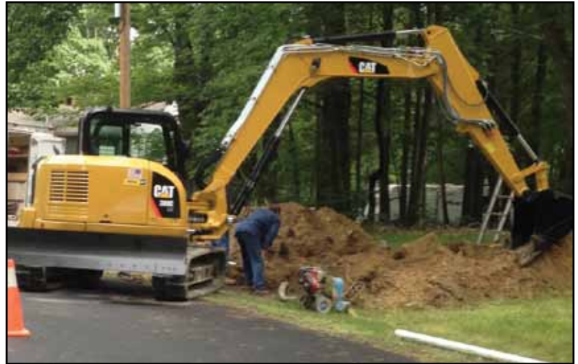
Excavation underway to replace water service connections.
