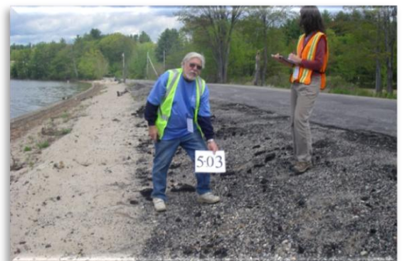
Bare, exposed soil, and runoff from the roadway on Rt. 153, results in delivery of nutrients and sediments into Province Lake. (Photo: AWWA)
