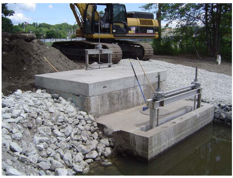
Figure 1-2. North Inlet Structure
