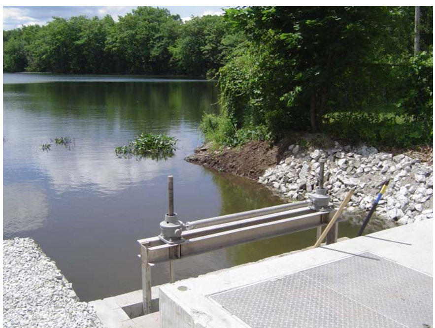
Figure 1-3. North Inlet Structure Looking Into Pond
