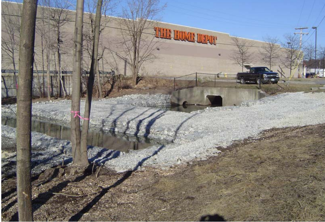
Figure 1-6. East Inlet Culvert Near Home Depot
