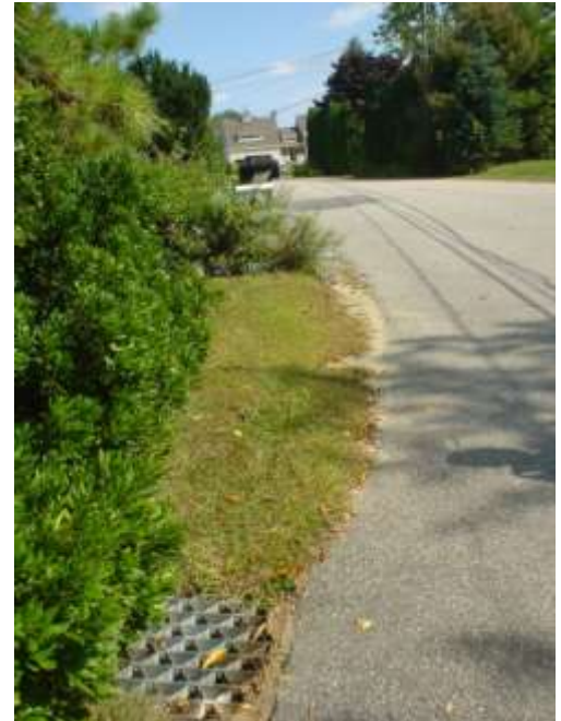
Basins catch stormwater that carries pollutants to Little River.
