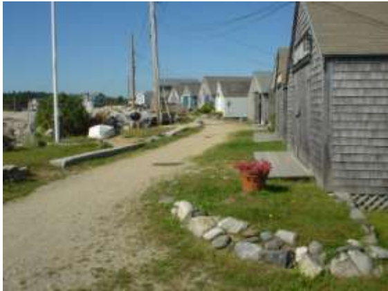
Seasonal cottages next to the Little River outlet have the potential to contribute a great amount of bacteria through sewage failures.
