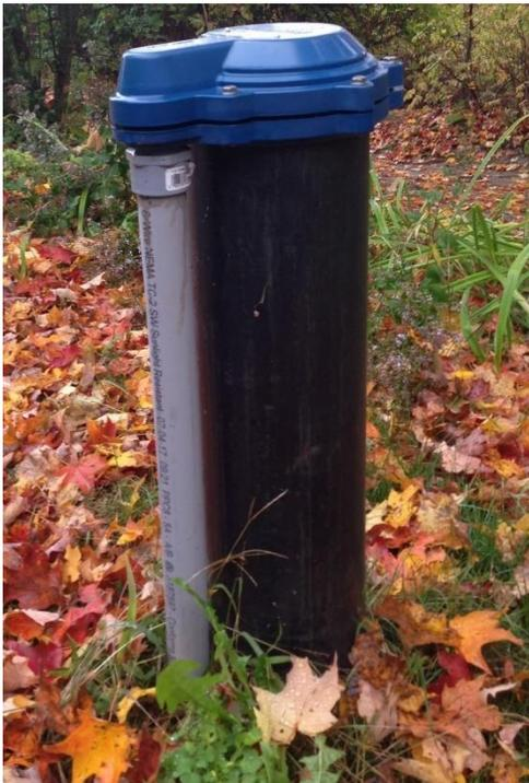
*A properly sealed wellhead*
