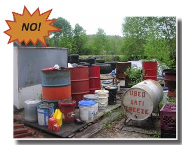
Antifreeze containers are in poor condition and some are open. There is no secondary containment to catch spills and leaks. These containers are not stored on concrete or other impervious surfaces to prevent leaks into the environment. They are exposed to the weather and should be under a roof.
