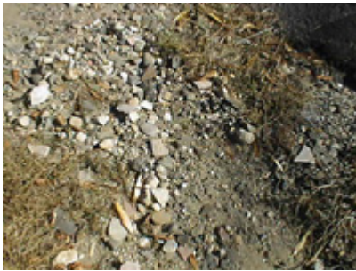
Asbestos sheet scrap scattered among small rocks
