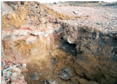
Red, white, and black baghouse waste uncovered while excavating a trench
