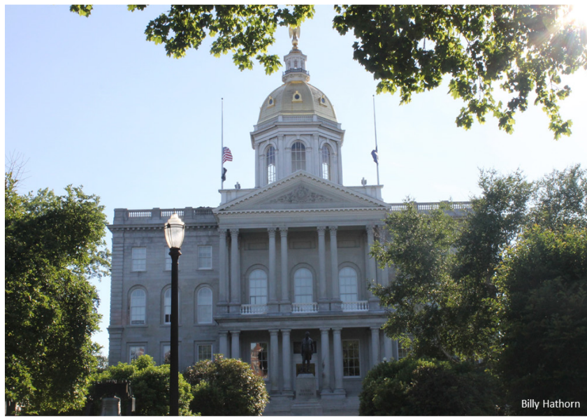
New Hampshire capital building
