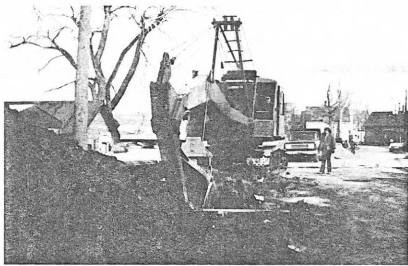
Above left: Seaward's Trackmobile hauls side-dumping RR cars full of gravel for backfilling a 60-inch sewer being placed as part of a $1.4 million contract.
