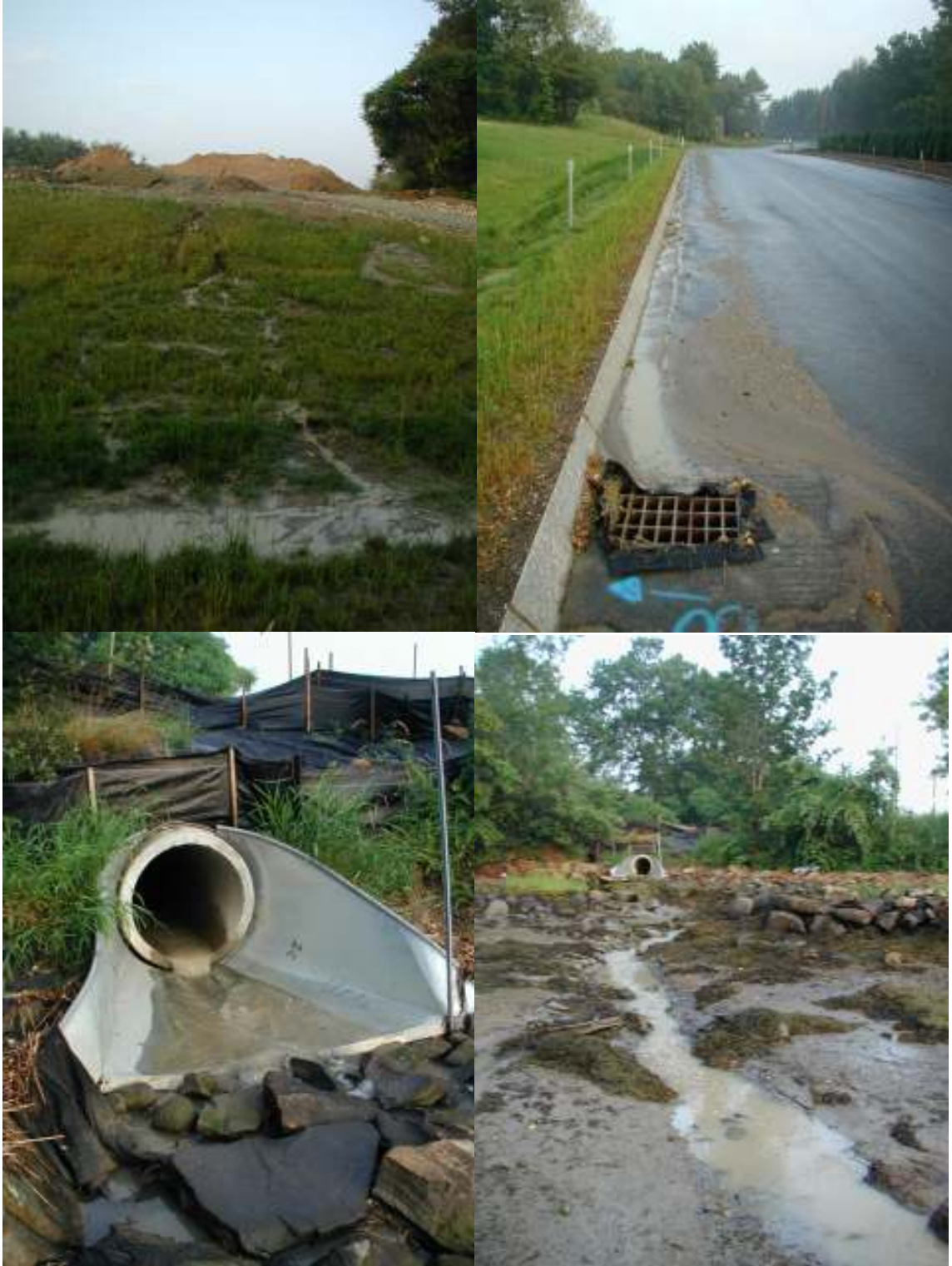
Figure 1: Run-off from highway and construction sites can be a major source of sediments. The above photographs were taken on July 11, 2006 in Newington, New Hampshire several hours after a rain storm. Sediments from a nearby construction site washed on to the surface of the road and into the storm drain system which discharged into Little Bay (Source: Newington Conservation Commission).
