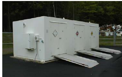
City of Keene’s permanent HHW facility storage container.
