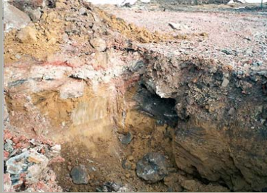
Excavation of asbestos with various waste types and colors.
