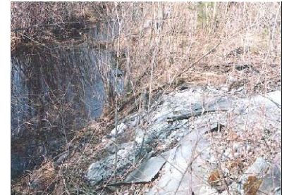
Asbestos wastes were used to fill this wetlands.
