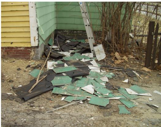
*Improperly removed asbestos from home renovation project.*
