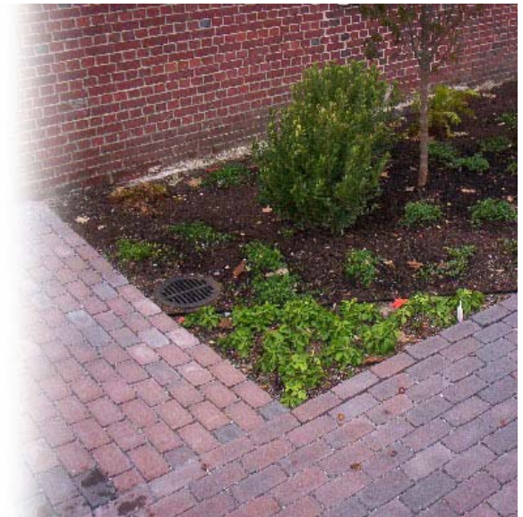
Rain garden and pervious pavement installation in downtown Peterborough, NH.
